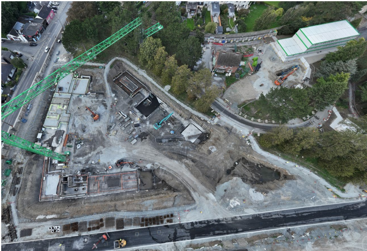
Picture taken from south direction showing New Infrastructure (Block 10)
