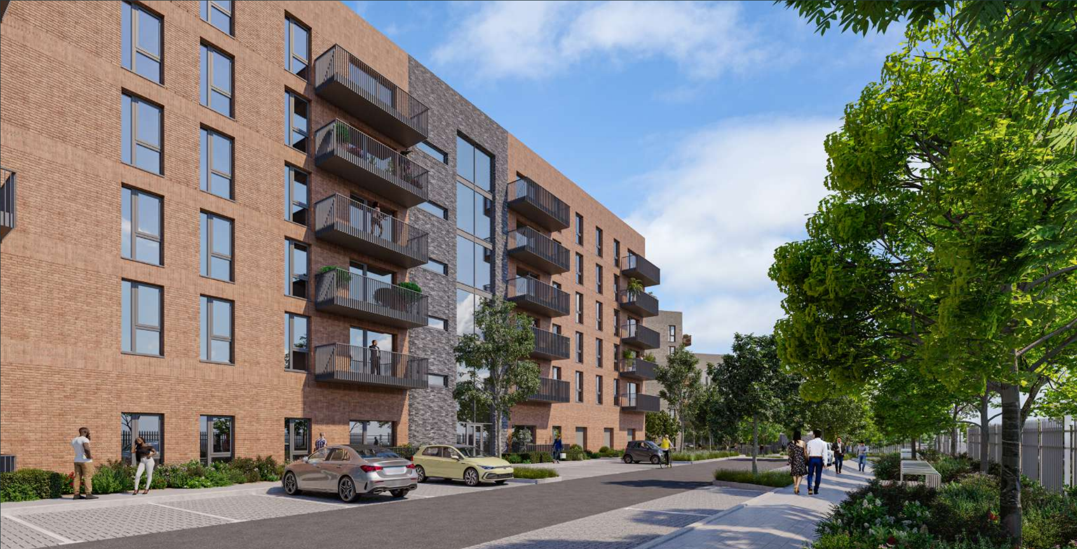
View from the Cookstown Road Entrance
