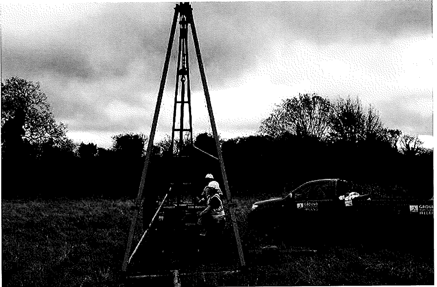
Cable Percussion Boreholing - used for Geotechnical and Environmental ground investigations.
