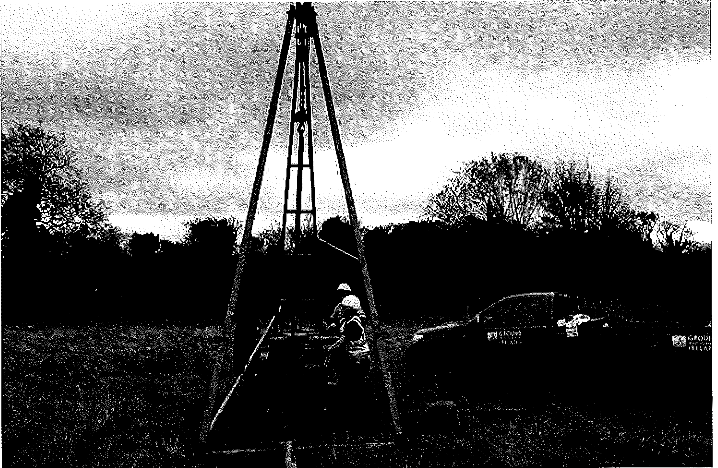
Cable Percussion Boreholing - used for Geotechnical and Environmental ground investigations.
