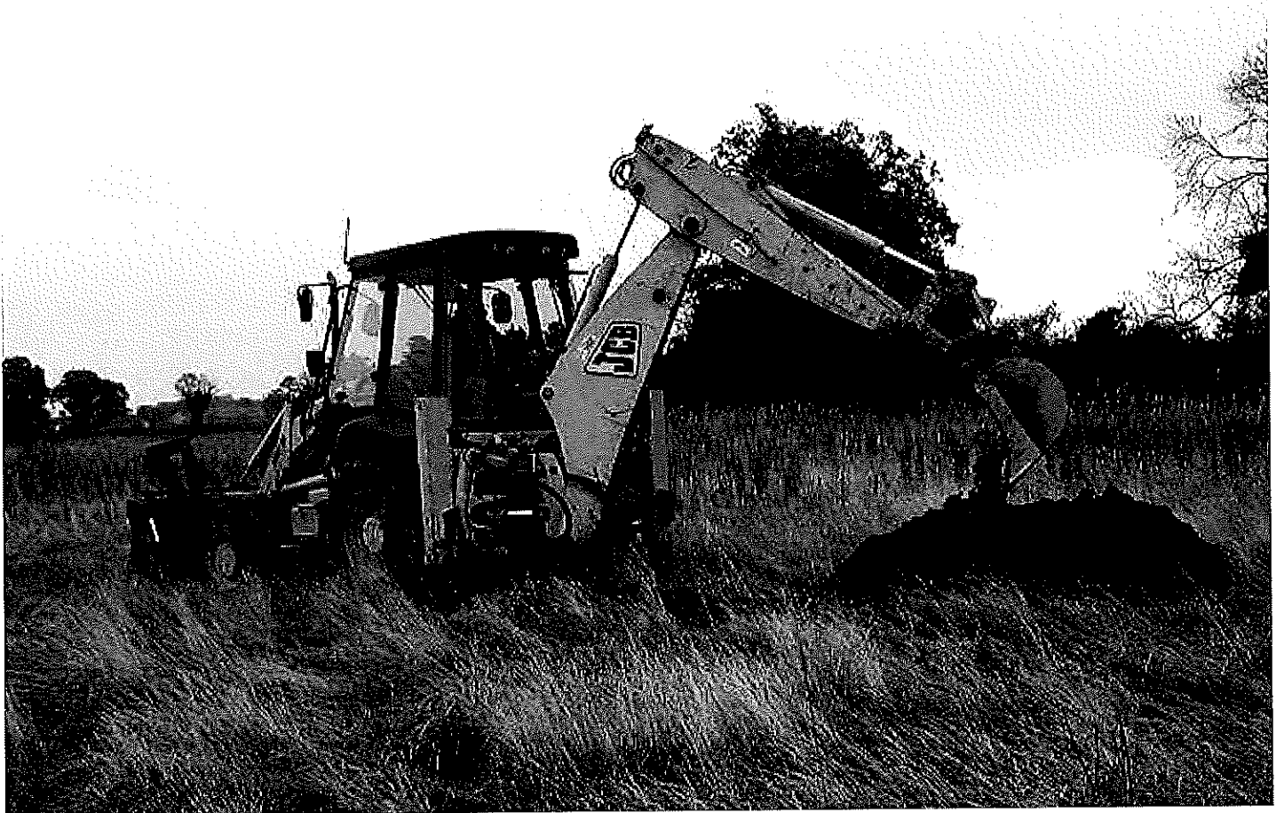
Trial Pitting – excavator required and allows subsurface soil types and relative thicknesses to be accurately recorded.
