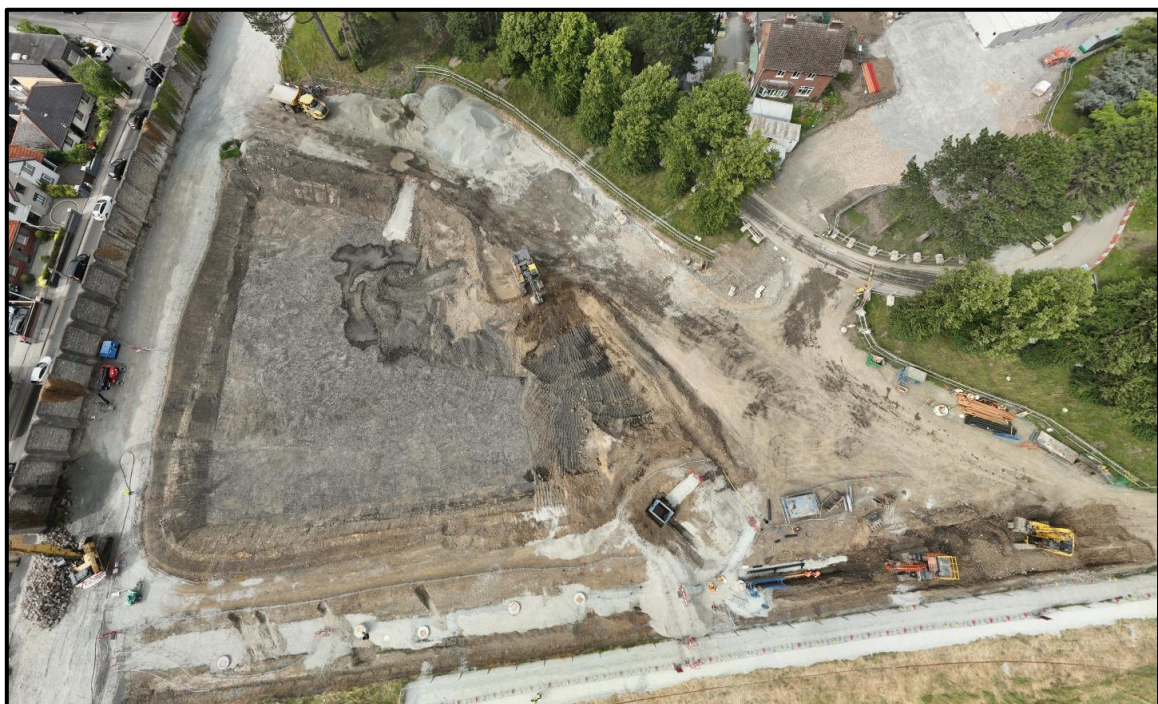
Picture taken from south direction showing New Infrastructure (Block 10)
